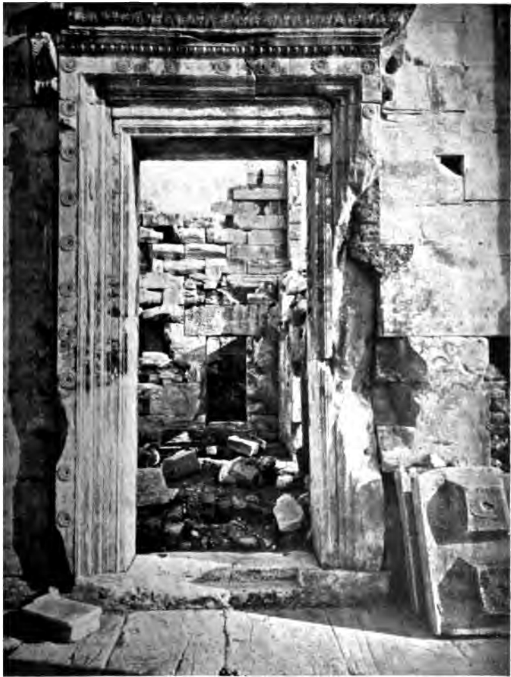
DOOR OF NORTH PORCH (before restoration) Erechtheum, Athens
